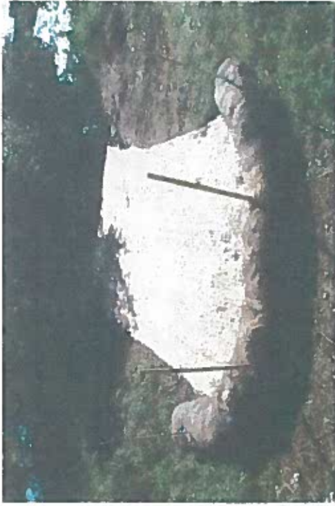
9 Area 4 after repair
